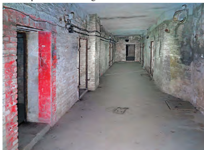
Corridor in Alexanderplatz bunker. Photo Clive Penfold
